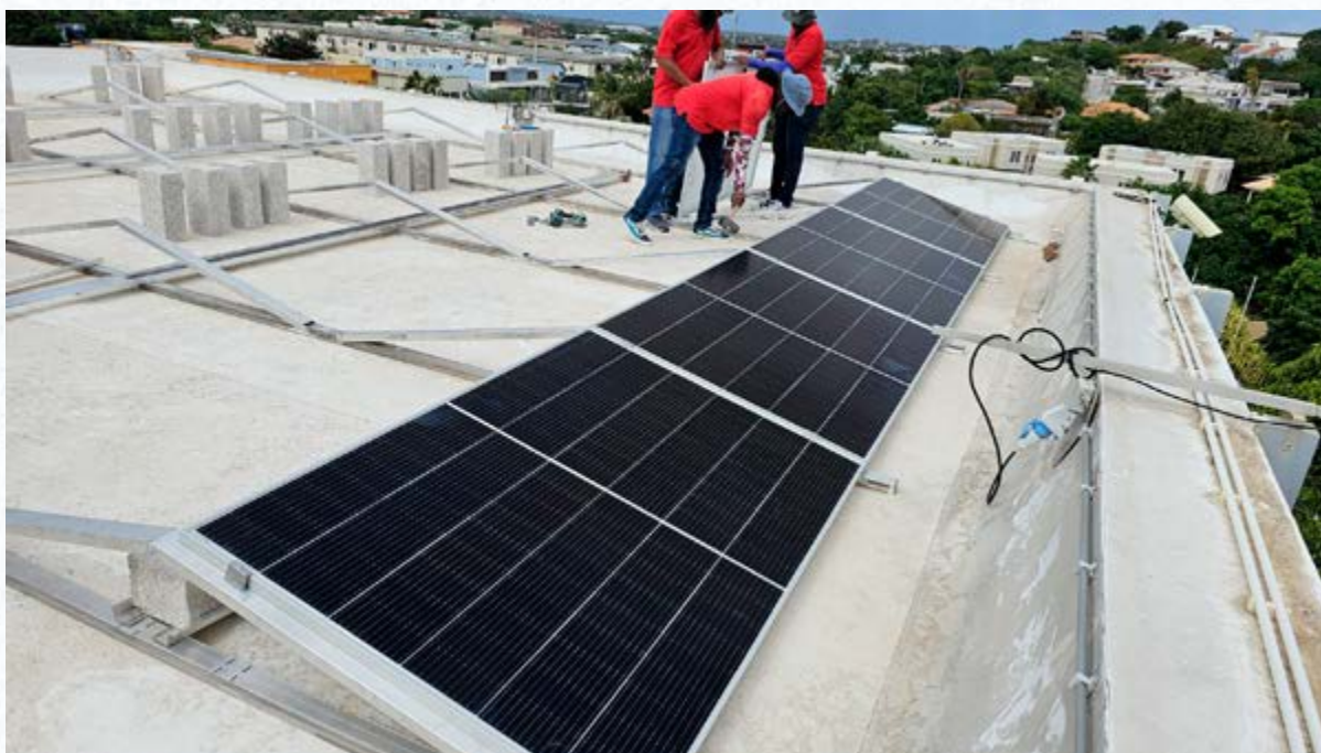
Solar panel installation underway at our Dutch Caribbean office.
